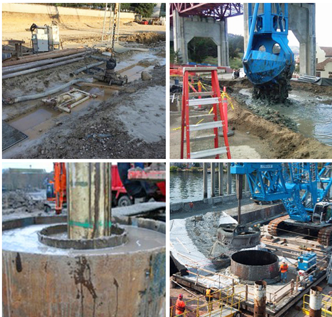
FIGURE 38 EXAMPLES OF CONTAINMENT MEASURES FOR A) TRENCH B) SPOIL C) CASING RESERVOIR D) BARGE
