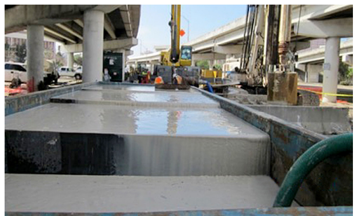
FIGURE 37 SEDIMENTATION TANKS FOR PHPA POLYMER DRILLING FLUID
