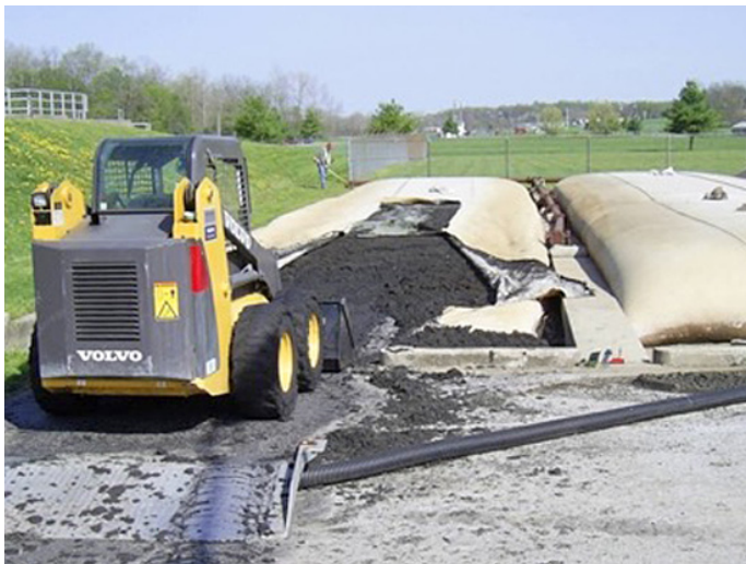
FIGURE 42 FILTRATION BAGS FOR PASSIVE SLUDGE DEWATERING
